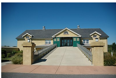
Front view of the DuPont dairy barn at BlueBall.
